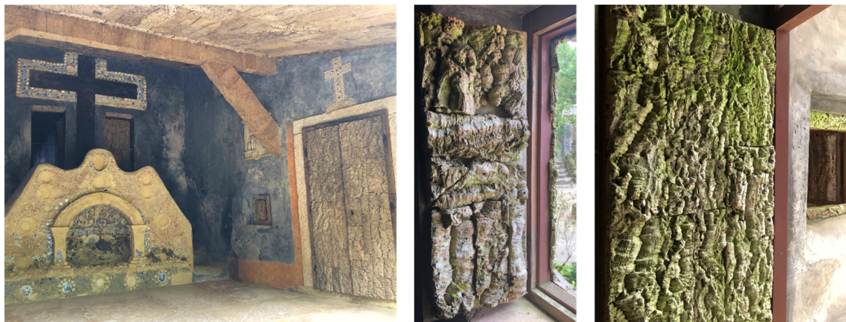
Figure 6. Images of cork use in the Convento dos Capuchos (Serra de Sintra, Portugal) as outdoor door covering (left) and as internal door frames (right). The cork used is virgin cork. Photos by Helena Pereira.
