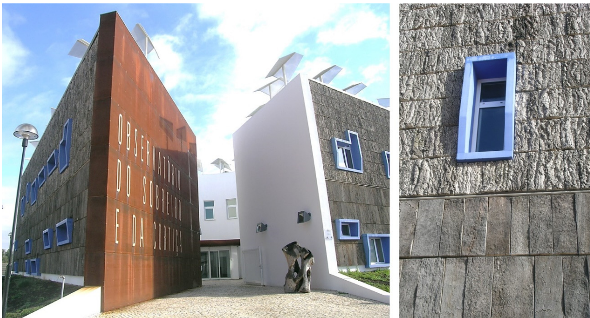
Figure 11. The Observatory for Cork Oak and Cork, designed by architect Manuel Couceiro, built in 2009 in Coruche, Portugal, with the façades covered by planks of reproduction cork on the lower part, and by pieces of virgin cork in the upper part of the façades. Photos by Helena Pereira.
