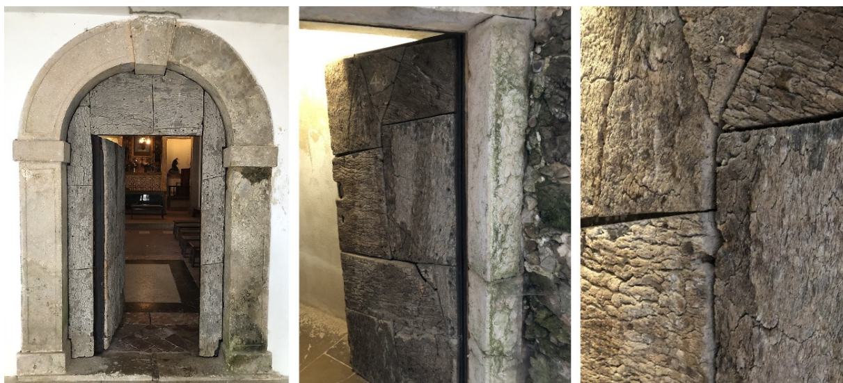
Figure 7. Images of cork use in the Convento da Arrábida (Serra da Arrábida, Portugal) as outdoor door covering to the chapel (left) using assembled cork planks of reproduction cork (right). Photos by Helena Pereira.
