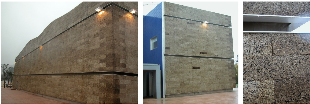
Figure 8. The Portugal Pavilion at Expo 2000 in Hannover, Germany, designed by architects Álvaro Siza and Eduardo Souto de Moura with façades covered by uncoated expanded corkboards, reconstructed in a city park of Coimbra facing the river Mondego, photographed in 2004 after two years of outside exposure after its 2002 construction. The NE façade is shown (left), as well as details of the uncoated expanded corkboards that were used. Photos by Helena Pereira.
