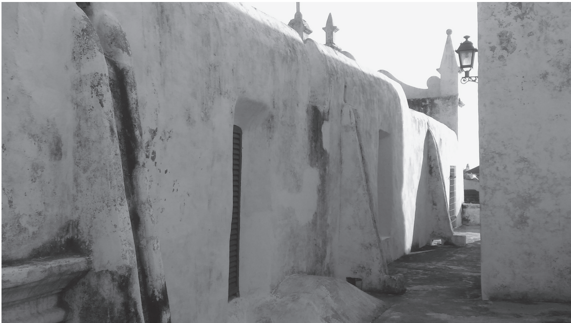
Figure 8.7 A pipe system on the Misericórdia terrace to conduct water to the cistern. Photo: Eugénia Rodrigues
