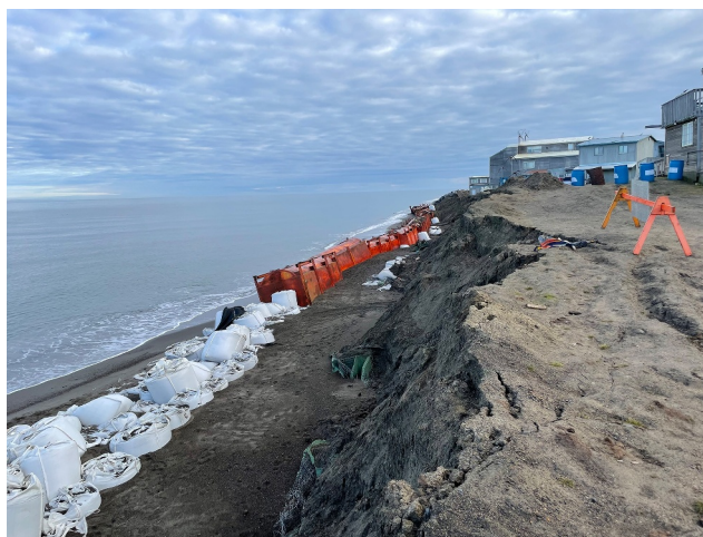
Figure A1. Example of rapid coastal erosion threatening coastal infrastructures at Utqiagvik (Barrow, Alaska). The photo was taken in September 2024. A road portion was destroyed after a storm during the summer 2023, we note the presence of red tanks and remaining big-bags down the bluff. Image credit: Benjamin Jones.
