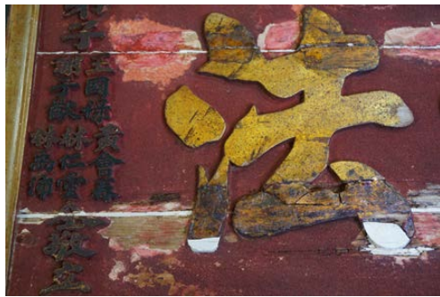
Fig. 8. Consolidated loose parts were then filled with Balsa Wood or calcium carbonate with acrylic resin Paraloid B72.
