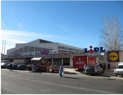
15.1964 Mercado Alvalade Norte Fig.48 http://www.cm-lisboa.pt/en/equipments/equipment/info/mercado-alvalade-norte
