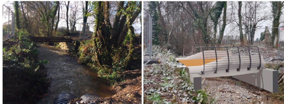
Figure A2. An existing structure on a greenway route at Roxborough, Midleton, Cork. A conceptual design of a blade bridge at the same location [44].
