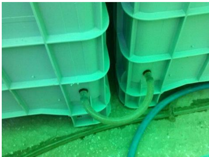
Photo 10: Particular of connection between 2 boxes
