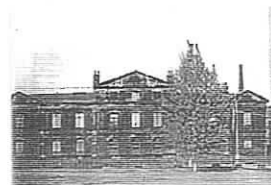
Fig. 92 O Globe Workes (1825), Green Lane, Sheffield pertencentes aos Ibotson Brothers. Edgar Jones, Industrial architecture in Britain (1750-1939) , London, 1985, p. 67
