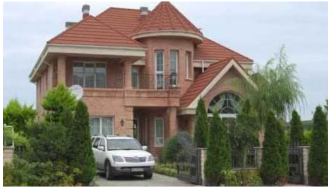
Figure 16 - A typical new home in the northern coasts and the Caspian Sea, photography of autor
