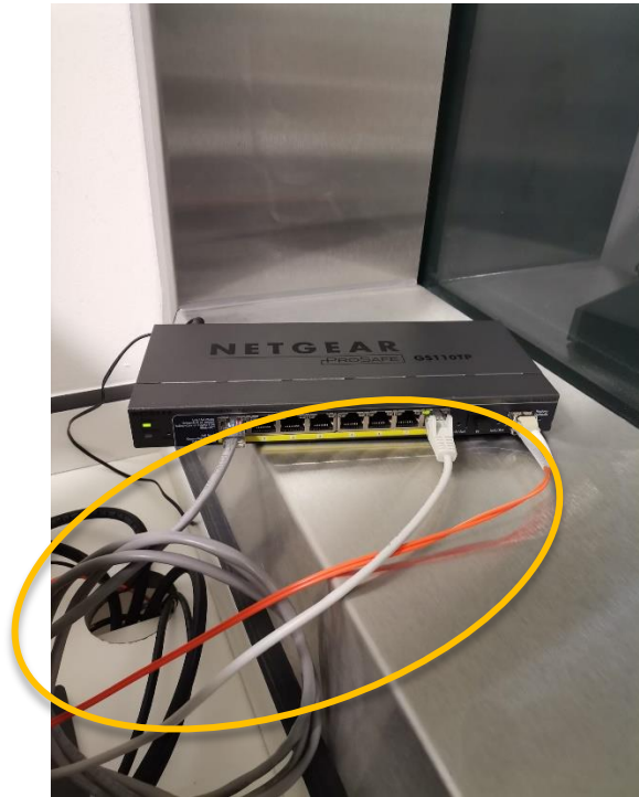
Figure 10.7: Fibre optic cables.
