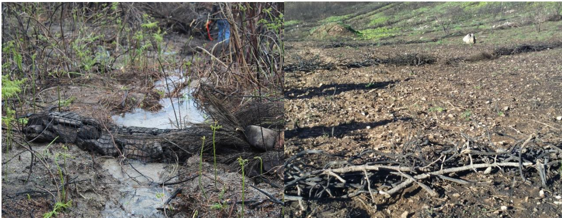
Figure 1.6 – Emergency stabilization interventions: rock check dam (left) and contour-felled logs (right). Both aim to detain runoff and sediments, decreasing soil losses after fire. (Photos by Luís Lopes)
