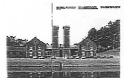
Station de Pompage do canal do centre
