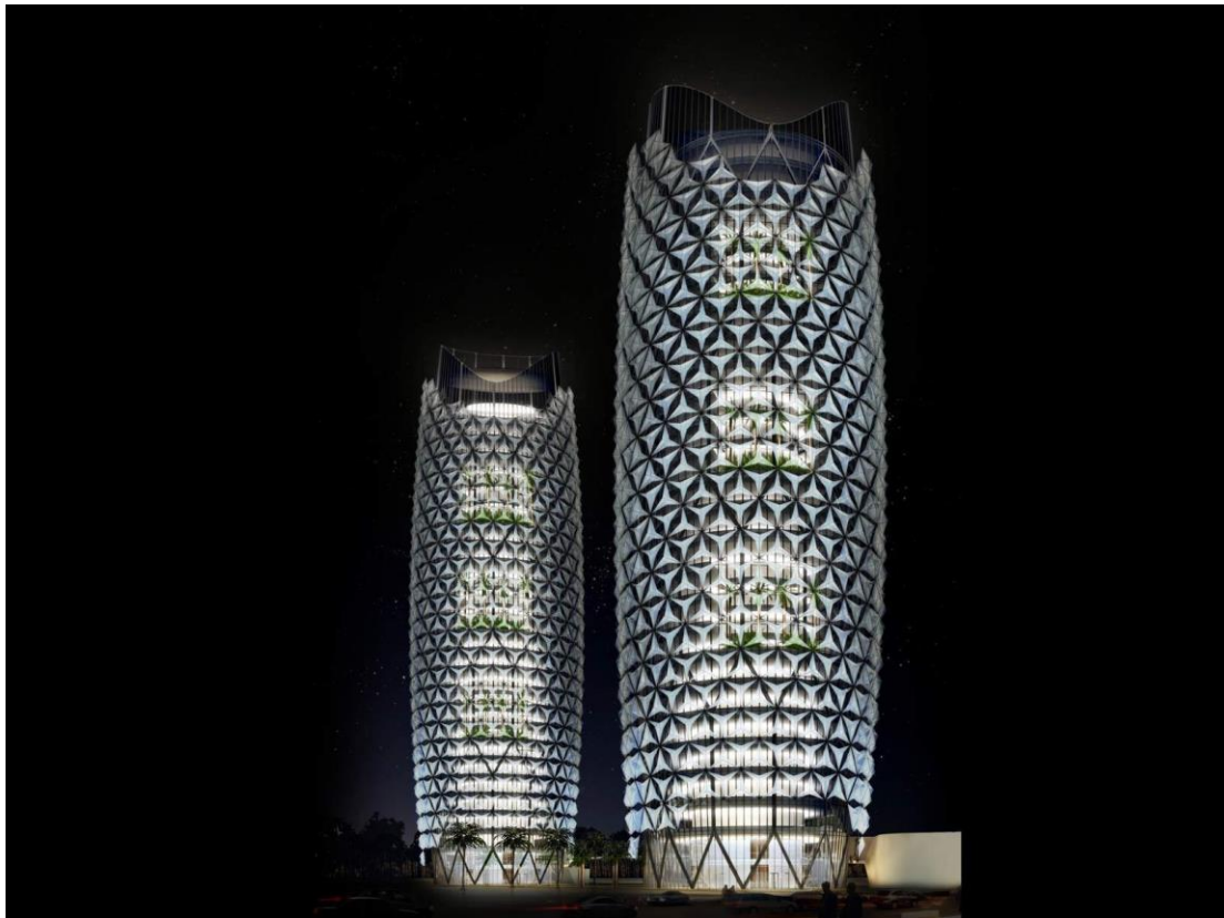
Figura 61: Iluminação noturna do Al Bahar (Fonte: http://www.archdaily.com/270592/al-bahar-towers-responsive-facade-aedas/ )
