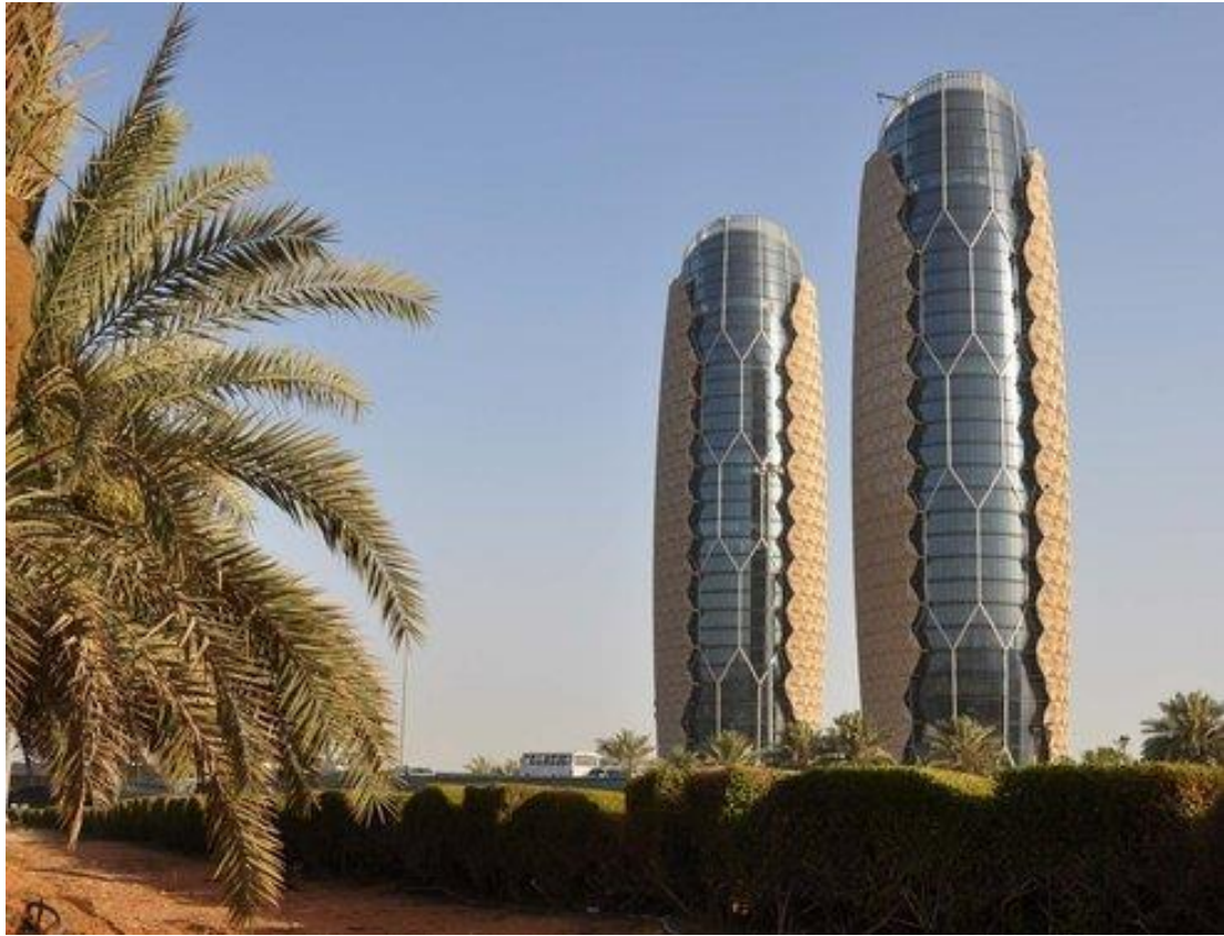
Figura 62: Fachada do Al Bahar (Fonte: http://www.archdaily.com/270592/al-bahar-towers-responsive-facade-aedas/ )
