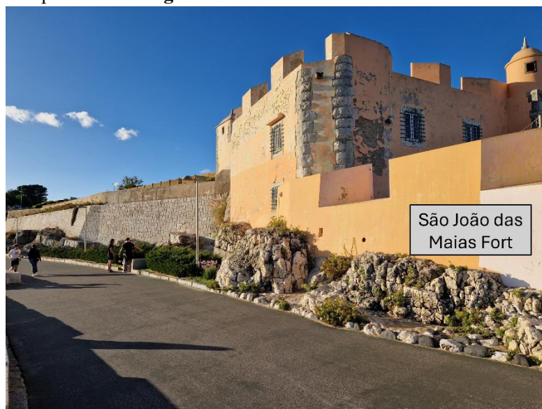
Figure 8.12 - Picture taken facing N where it is possible to observe that the Fort was built on top of the 3 limestone levels described before.
