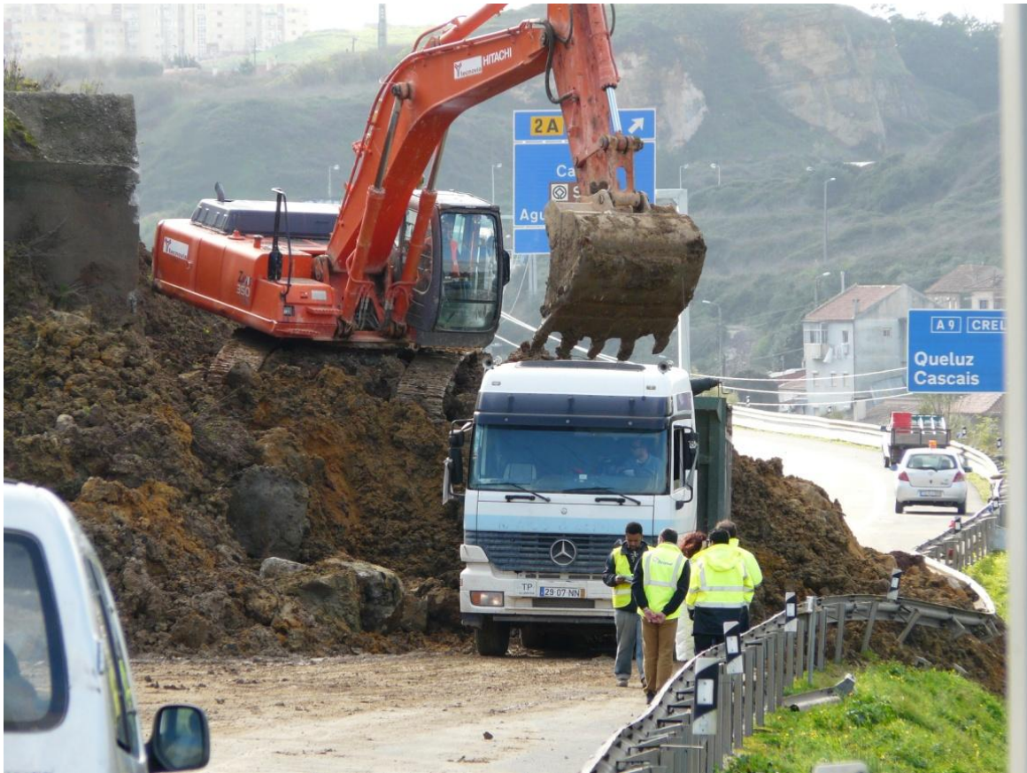
Fig. 0.2 - CREL interrupted by the landslide. Source: Sérgio Cruz de Oliveira, CEG, IGOT, Universidade de Lisboa, 24/01/2010
