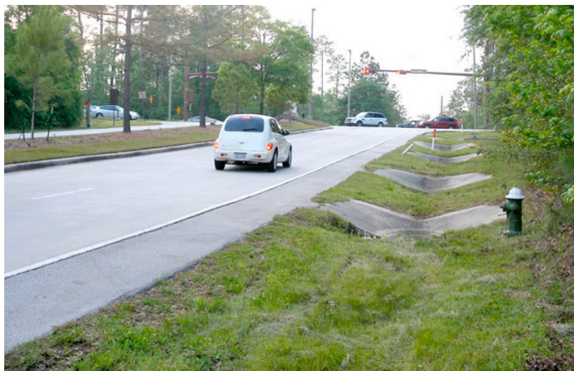
Figure 2.24 Open surface drainage at The Woodlands with check dams to retard runoff and promote infiltration where soils present good permeability (Yang et al., 2015)
