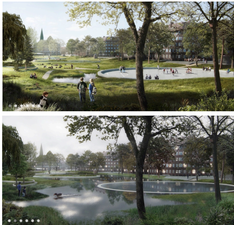
Figure 2.26 Render of the Hans Tavsens Park in 'The Soul of Nørrebro' project, showing the Park's temporary function as a rainwater retention basin ( www.sla.dk/en/projects/hanstavsenspark )
