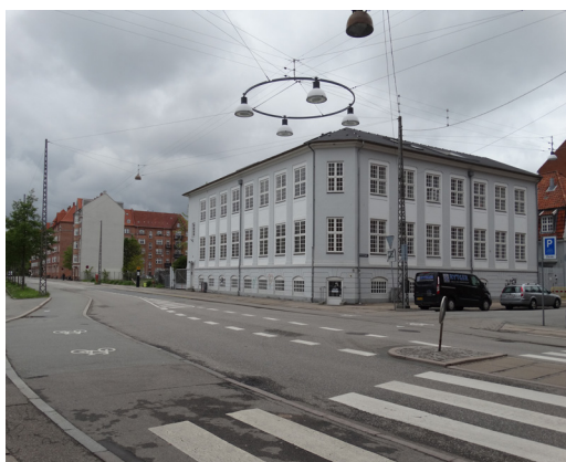
Ill.63 – Three-story existing office building.
