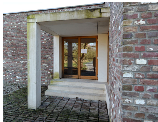
Ill.65 – Siza-Pavillon Insel Hombroich, Neuss-Holzheim by Álvaro Siza Vieira. Built in reclaimed bricks.
