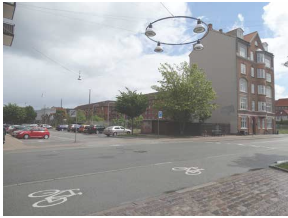
2021 | Unresolved facade of Sundholmsvej 57, facing Kornblomstvej Building
