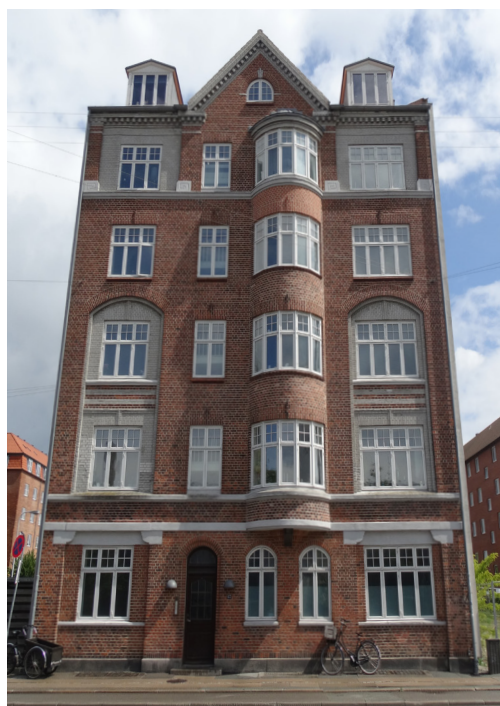
Ill. 48 – The existing building on the terrain, Sundholmsvej 57.
