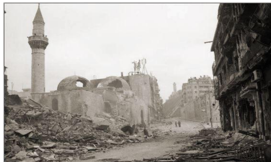
Figure 50: The destruction of Aleppo historical city-center. Source: UNESCO
