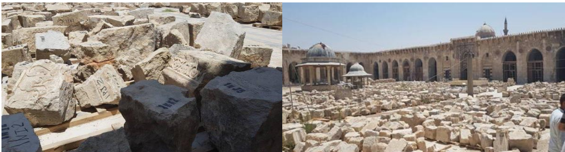
Figure 55: The historical stones, labeled and preserved for the reconstruction process in Umayyad Mosque. Source: Monia Faraj. Date:2018.
