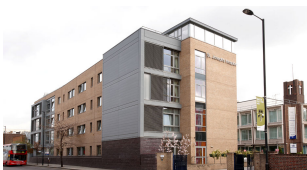
Fig. 11 | St. Joseph's Hospice ( http://salixmechanical.com/projects/health/st-josephs-hospice-new-community-areas/ )
