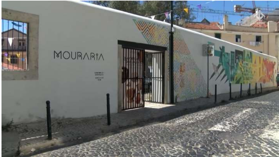
Image 108 - The Mouraria Innovation Centre's facade and ongoing construction in the background
