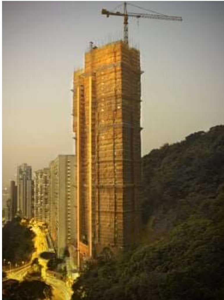
Image 49 - Bamboo scaffolding in Hong Kong (The Guardian, 2018d, picture is from 2009)
