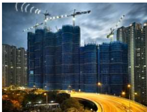
Image 48 - Bamboo scaffolding in Hong Kong (The Guardian, 2018d, picture is from 2008)
