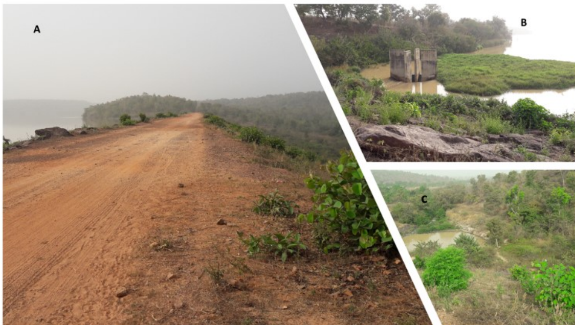
Figure 4:3 Doma Dam Project: (A) Dam crest; (B) spill-way inlet (C) Downstream outlet. Source: Daniel Adayi
