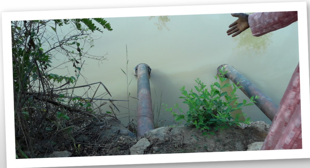
Figure 5:9 Mr Kindiri shows the intake point of the Doma irrigation structure that needed repairs for the GYES launching demonstration. Source: Daniel Adayi
