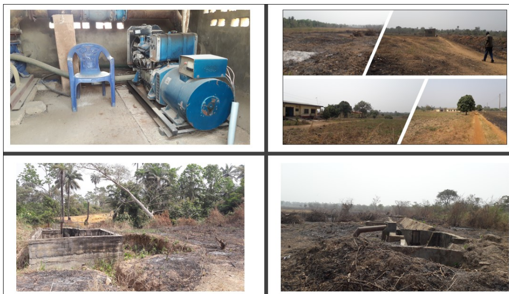
Figure 4:7 Oforachi Irrigation Project. Top (left) Power generator; Right: farmlands. Bottom (Left): chamber at the waterside; Right: the cement concrete trough. Source: Daniel Adayi.
