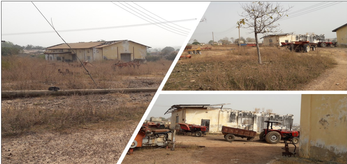
Figure 6:7 Pictures of Doma Project workshops. Courtesy: Daniel Adayi
