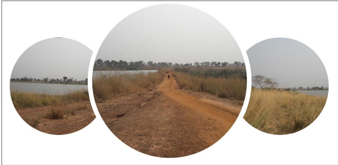
Figure 4:9 The Guma Earth Dam. Notice the footpath through the crest and the lush vegetation. Courtesy: Daniel Adayi.
