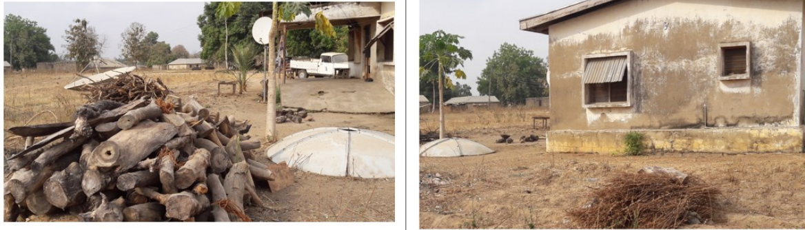
Figure 4:19 Front and side-views of the residential quarters of the Liaison Officer at Keffi. Source: Daniel Adayi
