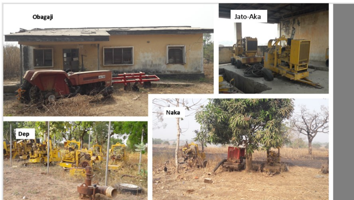
Figure 5:10 Abandoned power plants and tractors at the LBRBDA projects
