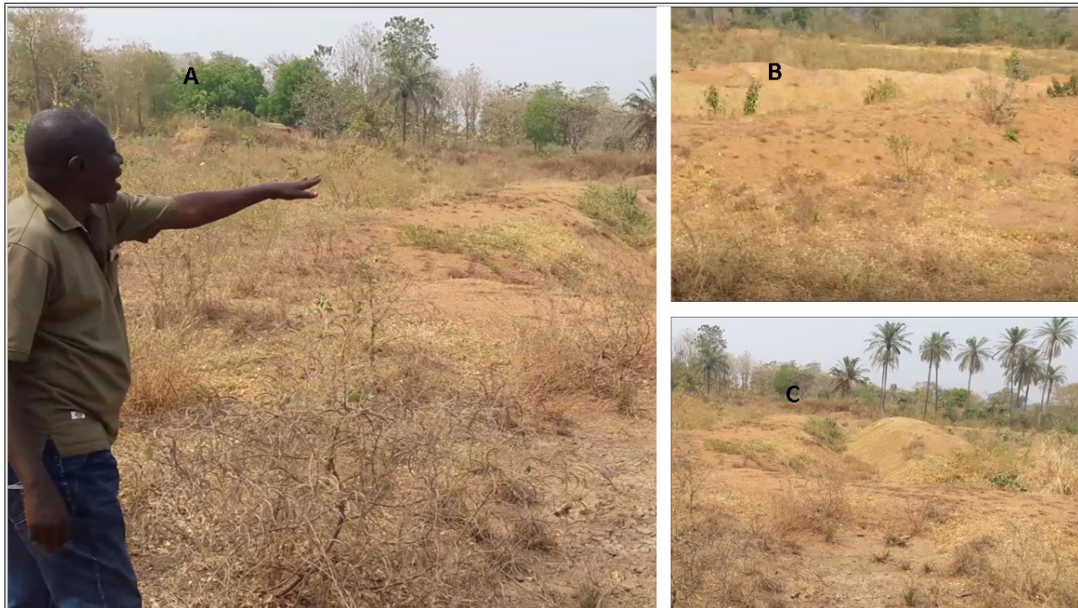
Figure 4:6 Oforachi Project (A): The Manager, Mr Kya Ochenge, explains the mechanism of the repository. Left (B) latitudinal view & (C) longitudinal views of the abandoned project. Courtesy: Daniel Adayi.
