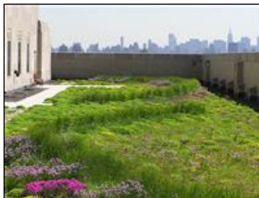
Figura 10 – Exemplo de cobertura extensiva, Bronx County Courthouse (Fonte: http://www.greenrooftechnology.com/extensive-green-roof )
