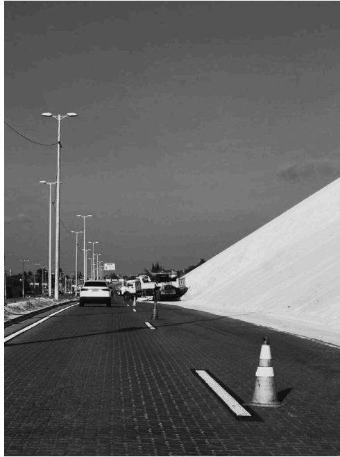
Figure 9.1 In spite of all the efforts to control them, dunes are still the best example of unstable environments: Dune of Sabiaguaba, Ceará, Brazil, encroaching on the road
