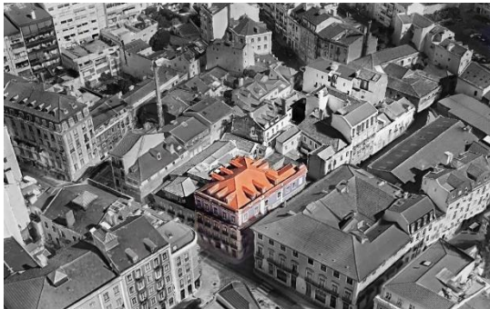
Fig. 7.1 – Fachada principal e lateral, quarteirão (Adaptado do Google Earth, 2022)
