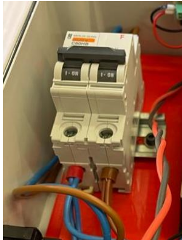
Figure 3-26 MERLIN GERIN MULTI9 C60HB 25844 B16 16A 16 AMP MCB C miniature circuit breaker.
