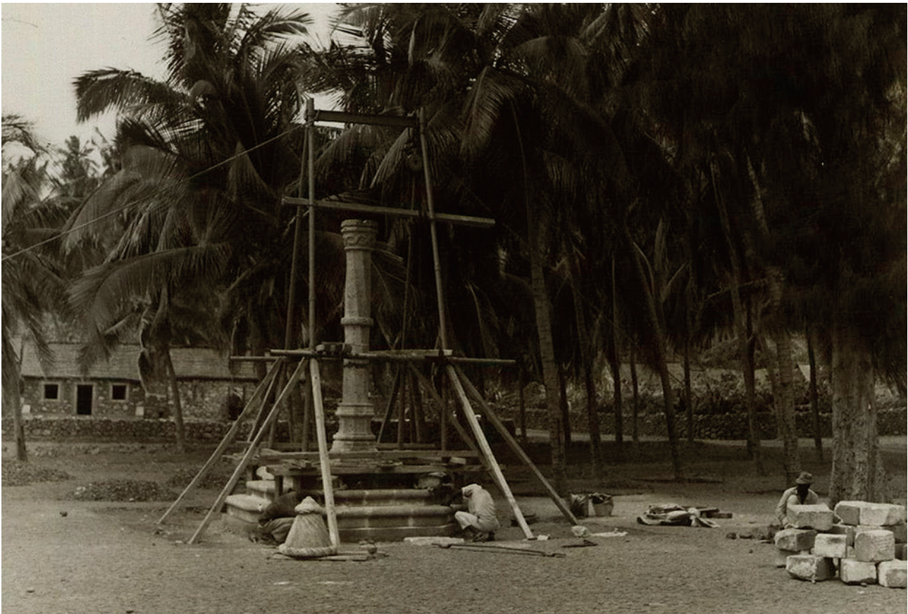
Fig. 12. Pillory of Ribeira Grande de Santiago (Cidade Velha, Cape Verde) during its restoration by Luís Benavente, 1970 (source: National Archive of Torre do Tombo, Luís Benavente collection, file 2085)
