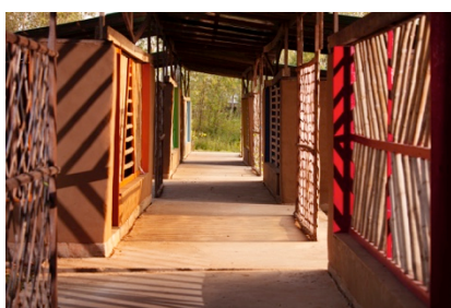
Figura 8 - Acessos entre as salas de aula da Kwel Ka Baung School.
