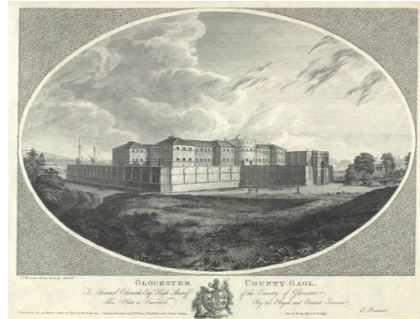
Fig. 30: The Gloucester County Gaol, s.d.
