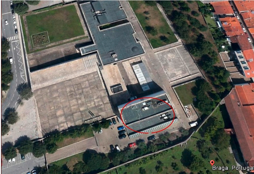
Fig. 1: D. Diogo de Sousa Museum, Braga (Google Earth). The structures with the mosaic panels are found in the interior of Block A.
