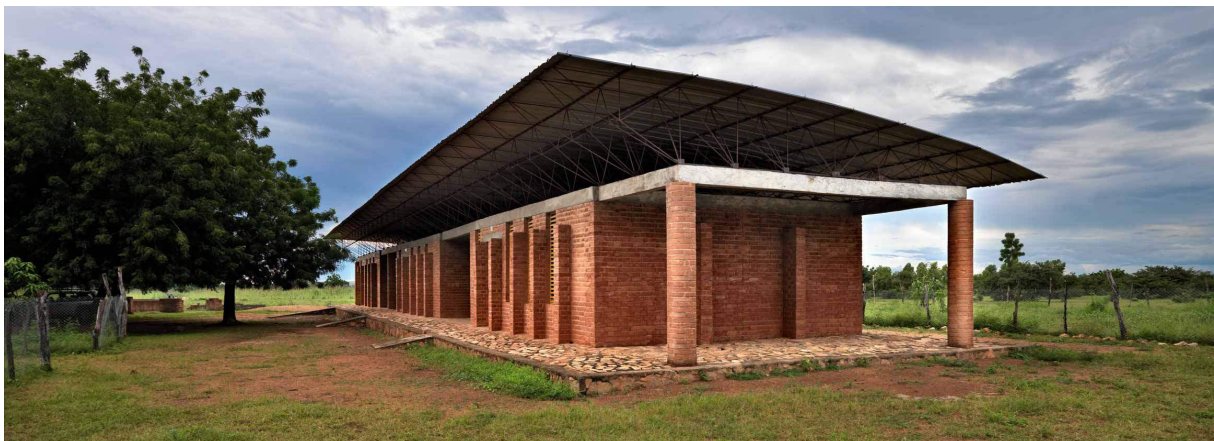
Figura 10 Gando Primary School
