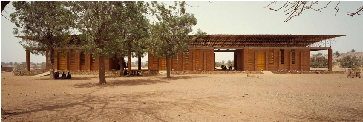
Figura 12 Gando Primary School
