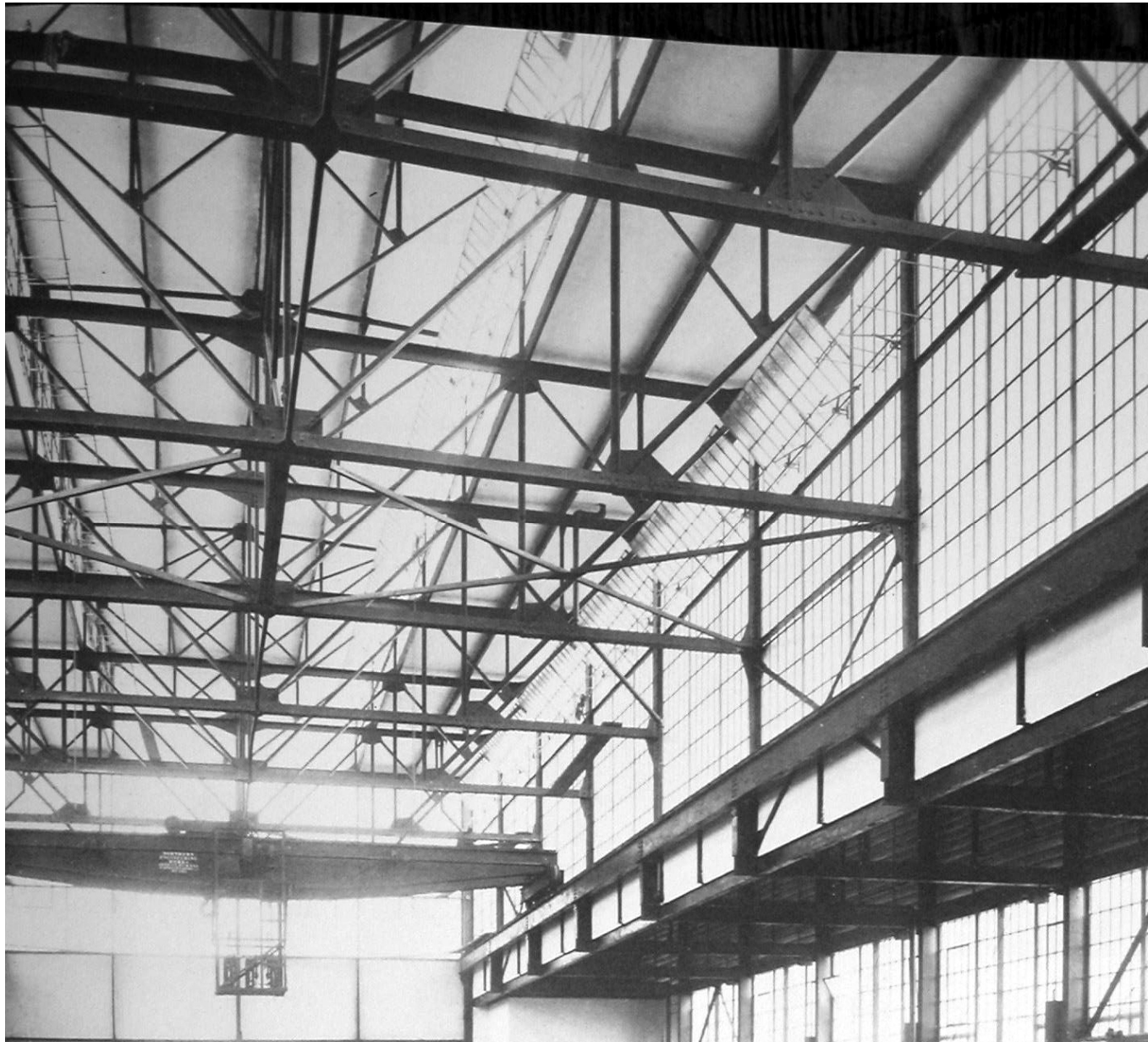
Fig. 5.32. O interior da Forge Shop (in The American Architect , 1911: 240). Fotografia de Manning Brothers.
