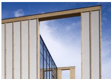
Fig. 57 Utilização da palha como preenchimento das paredes, The Gateway Building, Nottingham, R.U., Make Architects; http://assets.inhabitat.com/wp-content/blogs.dir/1/files/2011/11/UoN-Gateway-Building-Make-Architects-3.jpg
