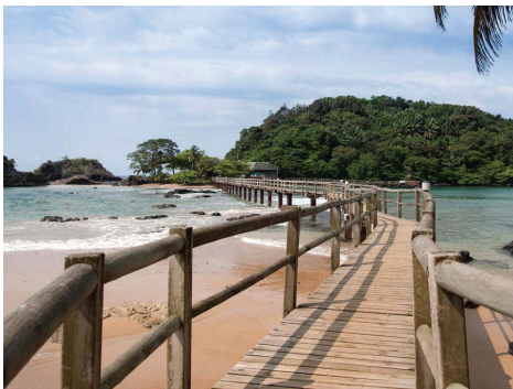
Fig 15 | Bom-Bom Island Resort - Príncipe | https://destinia.pt/h/h377936-hotel-bom-bom-island-resort
