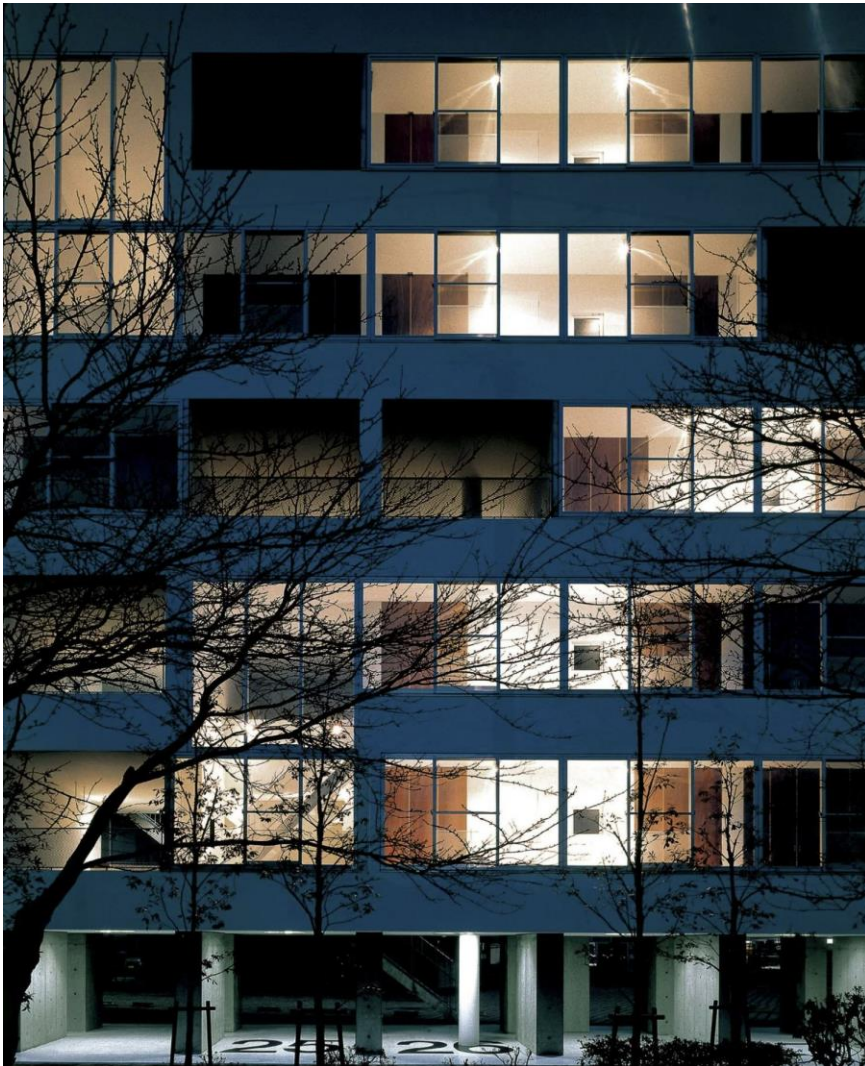
26. Fachada Sul do Kitagata Apartment Building.
