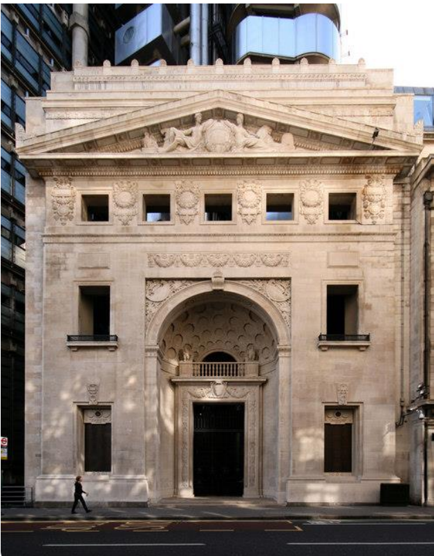
19. Fachada existente conservada no Lloyd's building.
