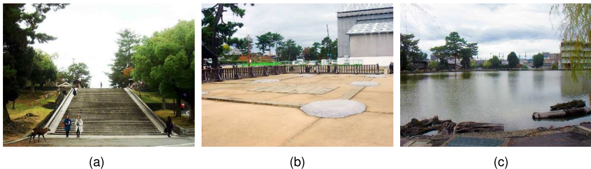
Figure 11 – Tōfuku-ji Temple - (a) Entrance staircase at Tōfuku-ji Temple: “At the entrance there is a beautifully built stone staircase, and on each side of the door, two giants of astonishing height with maces in their hands.” (Fróis, 1565); (b) foundation stones of the entrance gate: “It has a door about 40 feet high and 5 feet wide; with columns of two fathoms in thickness.” (Fróis, 1565); (c) Sarusawa-ike pond – “Outside the main entrance there is a pond fifty fathoms long and fifty fathoms wide, which is brimming with fish that no one dares to fish” (Fróis, 1565) (Photos by author)
