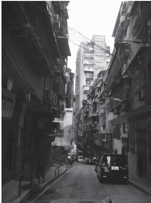
Fig. 7 — The Steep Alley at Santo Agostinho
