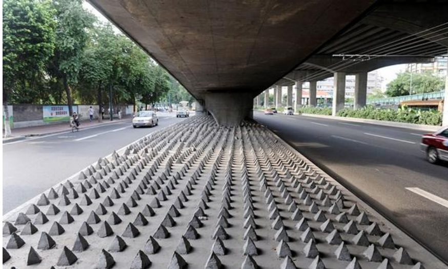
Fig.9 “Concrete spikes under a road bridge in Guangzhou city, Guangdong, China.”
