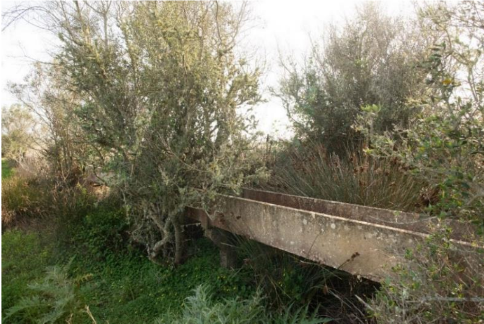
Fig.16: raised cement aqueducts. Abicada, 2020
