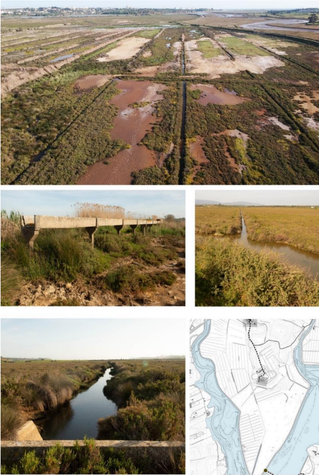
Fig. 55: Channels, Ditches, Aqueducts from the Agricultural Development Works
