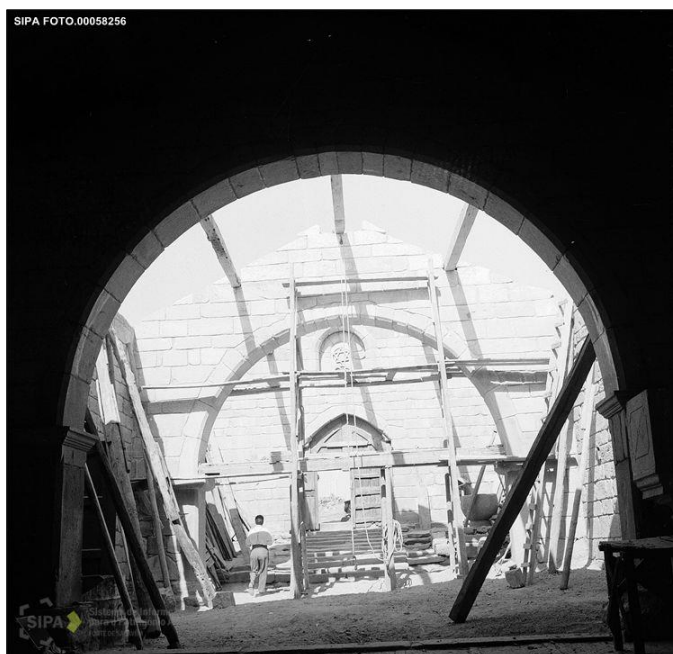
Fig. 89 Interior durante as obras © IHRU: DGEMN/DSID IPA.00002120
