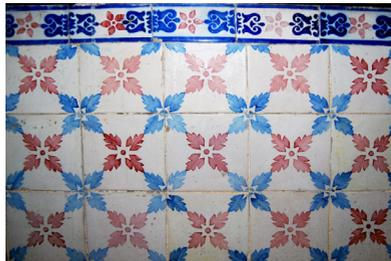
**Figure 16.** This beautiful flower pattern is unknown from façades and was likely made for interiors. The chequered application of small tiles (called “lambrihas” in Portuguese) on both sides of the sill was used by Roseira, in the 1860s and 1870s, for the detailing of small areas including shop fronts, in black and white, blue and white, or yellow and white. They were later replaced by full-sized tiles, each with a number of squares rotated by 45°.
