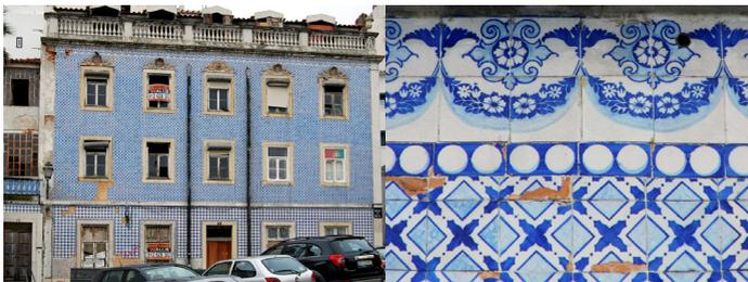
**Figure 12.** House of João Roseira in Beco do Belo (photo taken on November 2012 by Lurdes Esteves). The second-floor windows are decorated with ceramic pediments simulating carved stonework, carefully encircled by the frame tiles, some of which are uniquely shaped to fit the pediments. This floor was the noblest in the house and may have been inhabited by the proprietor and his family.
