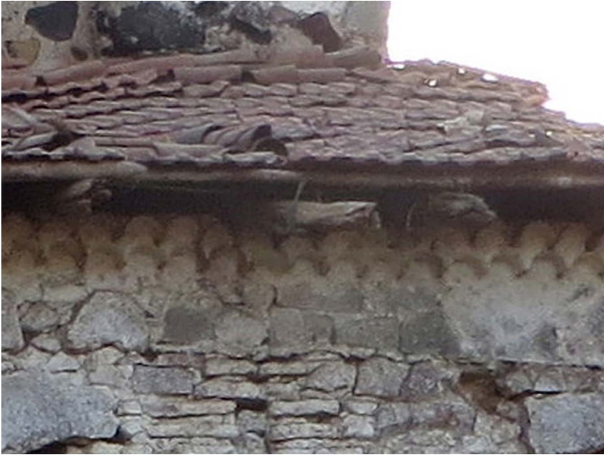
Image 16 – Fortified manor house of Dongaripada, roof with a Portuguese-type double eave (photo: Joaquim Rodrigues dos Santos)
