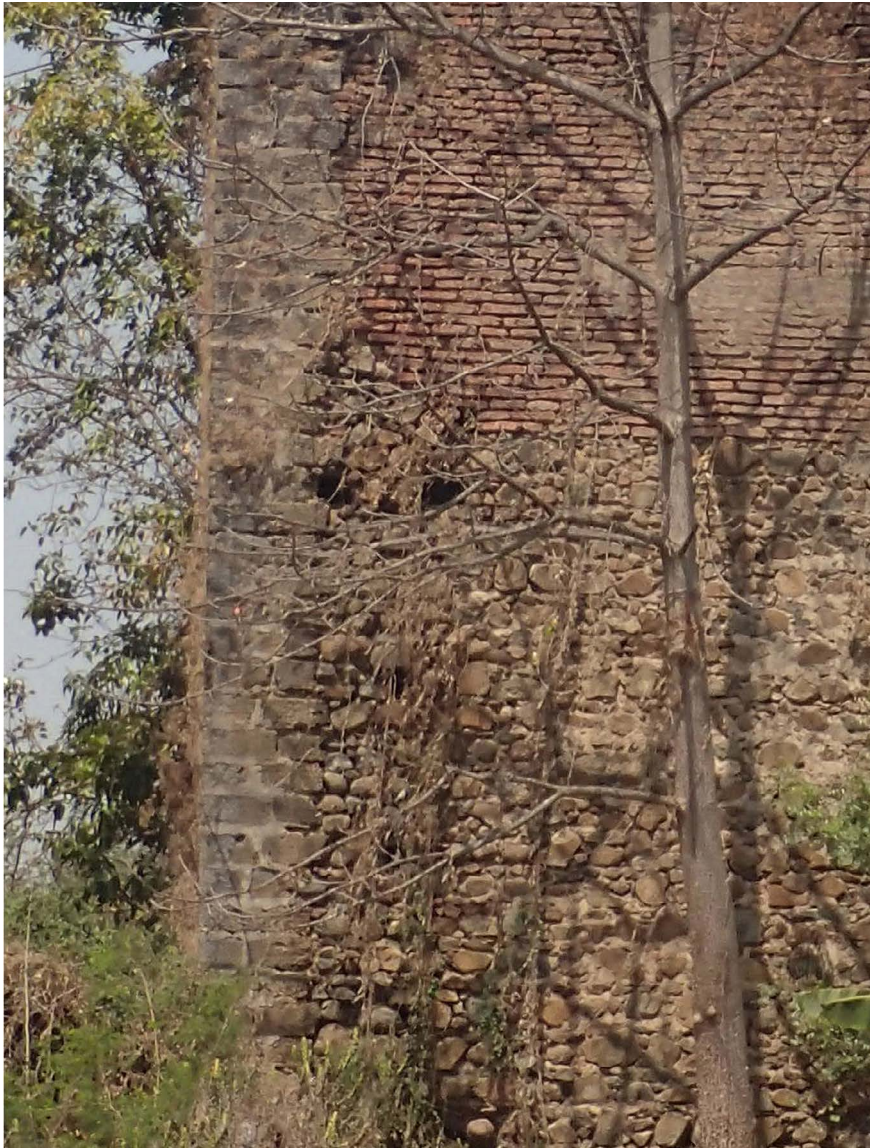
Image 14 – Fortified manor house of Solsumba, with a brick masonry wall on the upper floor, resting on irregular stone masonry
