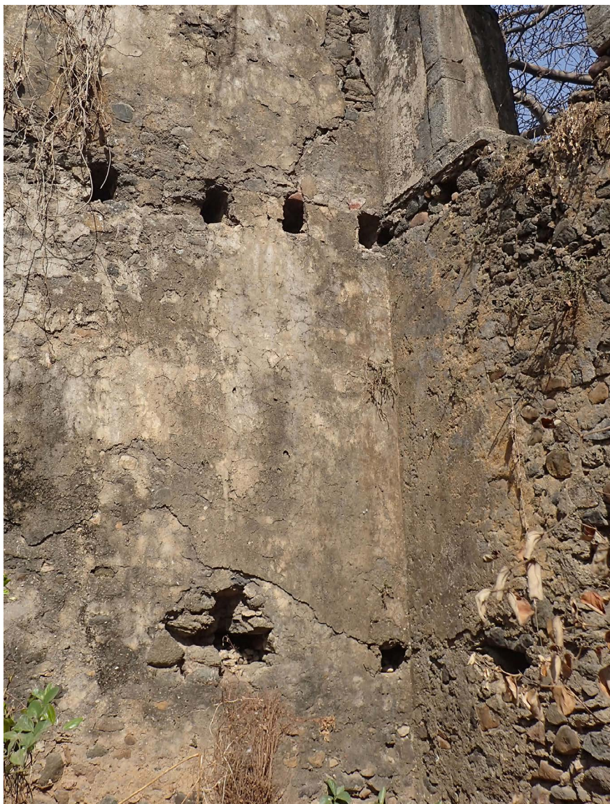
Image 17 – Fortified manor house of Kalgam, holes of wooden beams found in the ground floor ceiling ( photo: Joaquim Rodrigues dos Santos )
